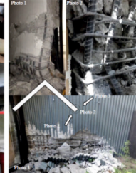
Figure 4: Lateral irregularity resulting in one-storey beam-column joint and column. (a) transfer beam right and damage; (b) transfer beam right and damage; (c) transfer beam right and damage.
