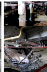
Figure 4: Lateral irregularity resulting in one-storey beam-column joint and column. (a) transfer beam right and damage; (b) transfer beam right and damage; (c) transfer beam right and damage.
