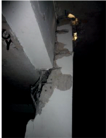
Photo 2-4 Damaged RC column
