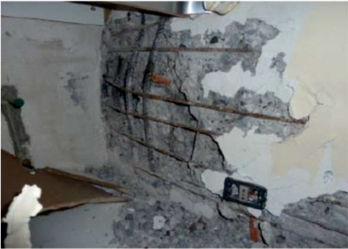
Photo4-3 Internal view of photo 4-2
