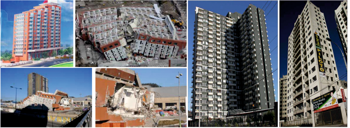
Figure 4.19 Alto Rio condominium in Cocepcion. structure toppled on one side, and failure of bearing walls
