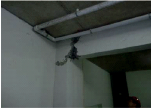
Photo4-4 Underground portion of photo 4-2
