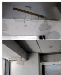
Fig. 3 Beam cracking in 22-story RC moment frame (precast cast-in-place)
