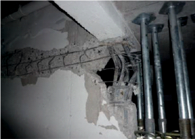
Photo 2-3 Close-up of wall column
